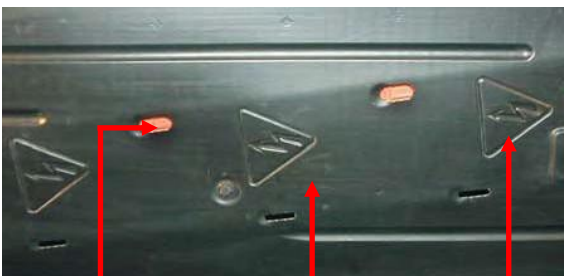
High-Voltage Cable Visible
